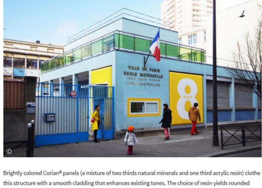
thermoformed angles that emphasize the joint, creating a slight floating back panel with the existing
